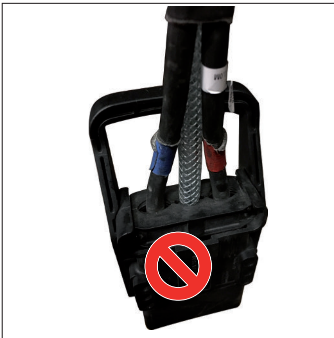
Fig. 34: Incorrect laying, fabric tube doesn't correspond to the requirements of the specification
